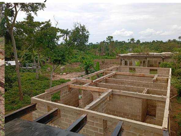
Omitide's building at the lintel level
