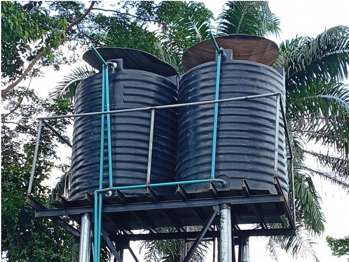
Rainwater Harvesting Kits installed on our demo farm
